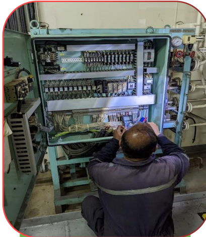
Ship Control Panel Repairs
